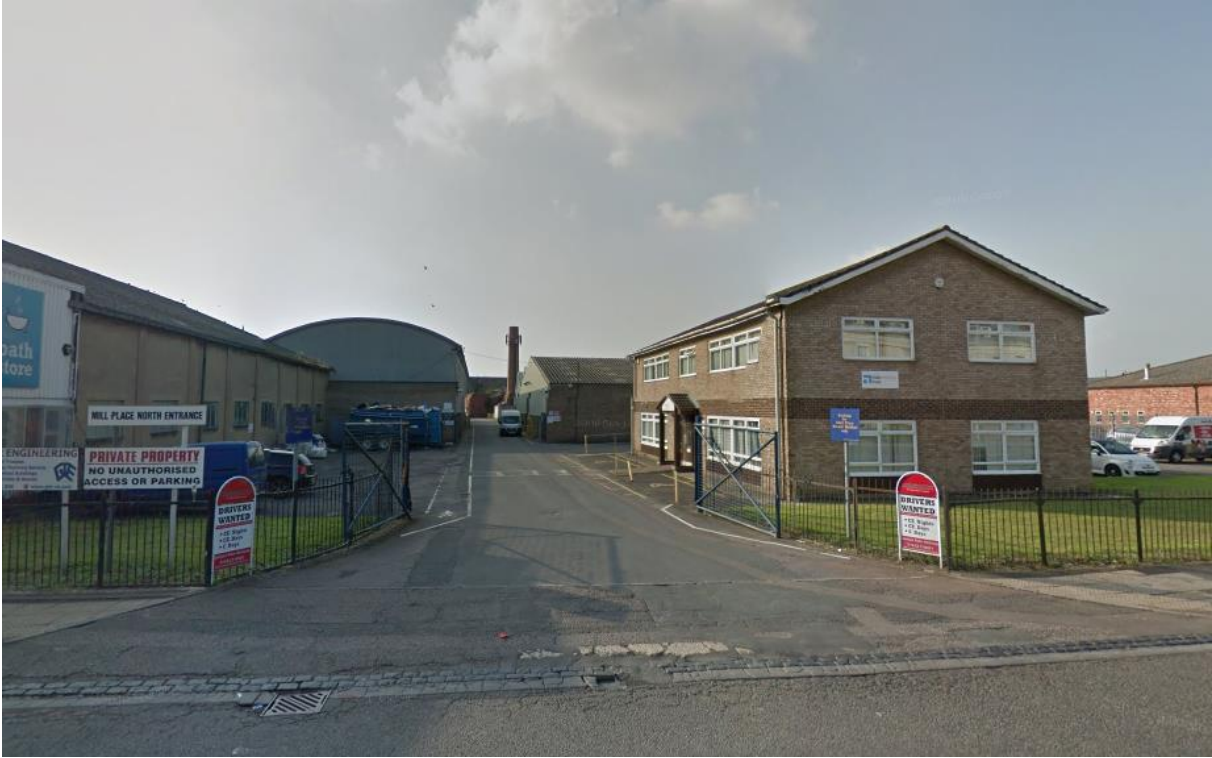
Plate 8 Madleaze Chimney from the east after height was lowered
