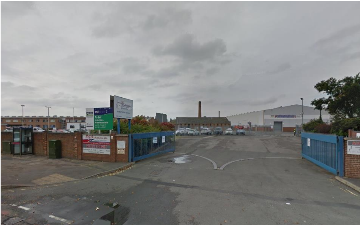
Plate 9 Mill Place Chimney from the east
